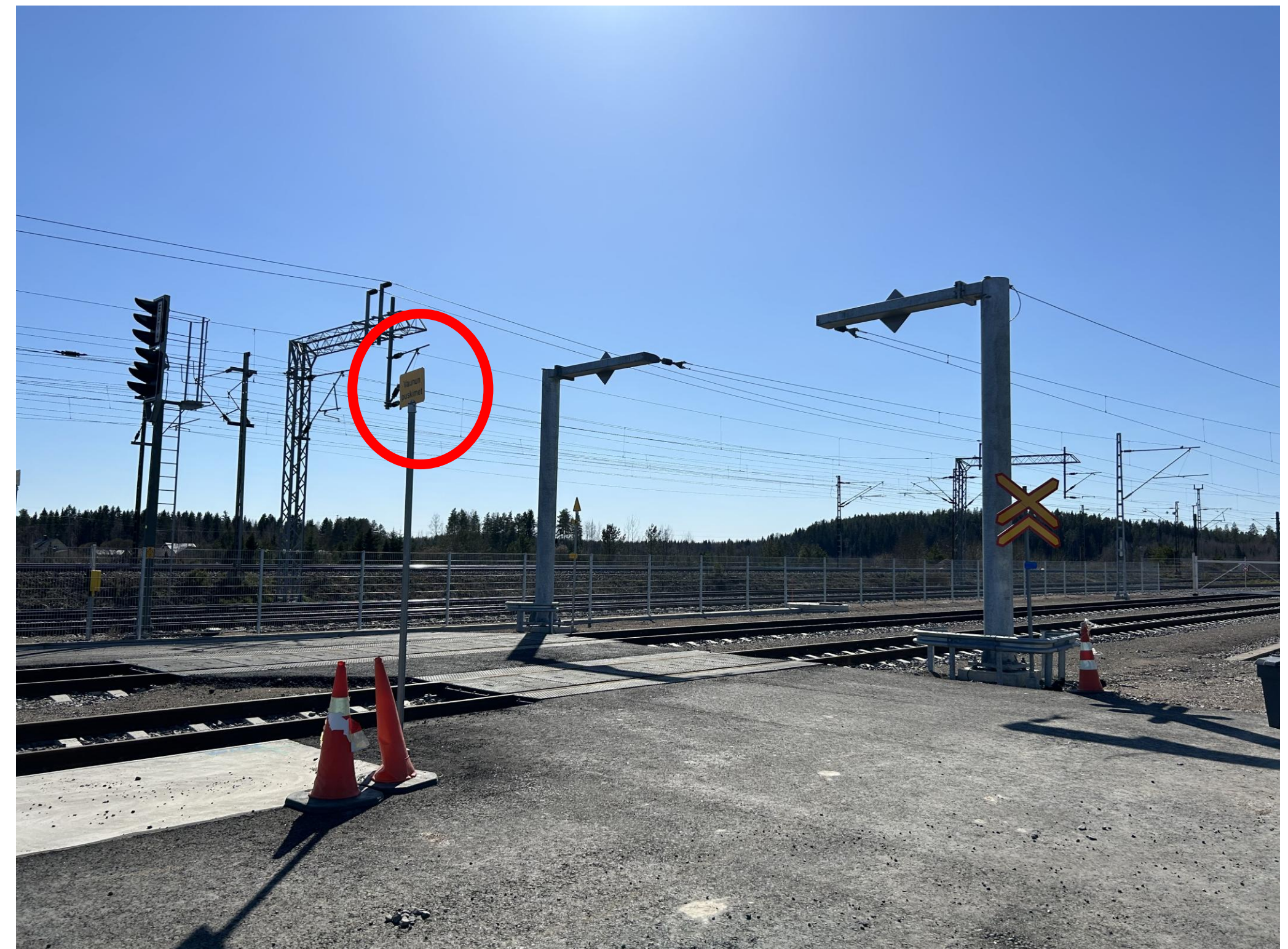
Track 907 alignment mark circled in the image.
